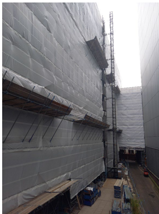
New union street – Scaffolding complete
