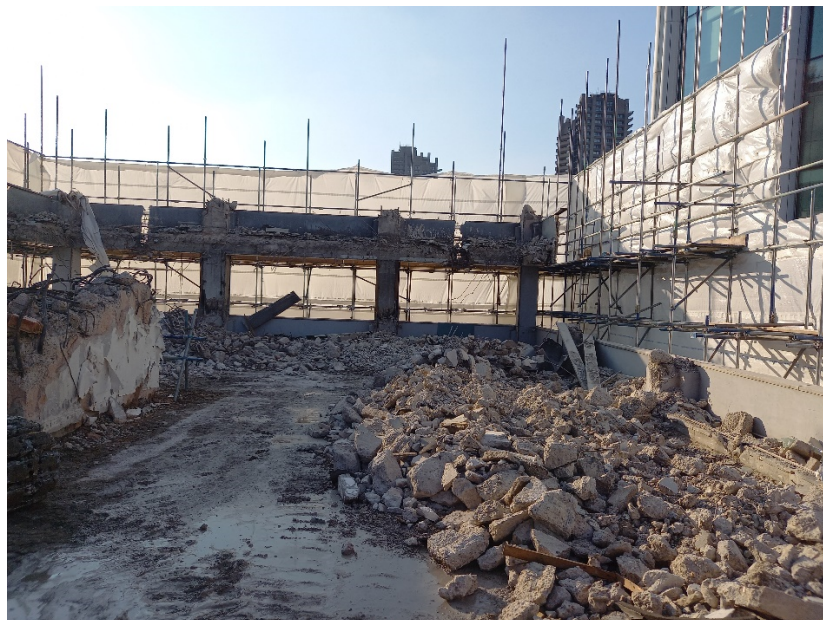
Typical floor demolition - level 9
