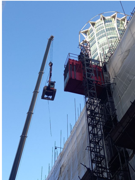
Excavator lift level 4
