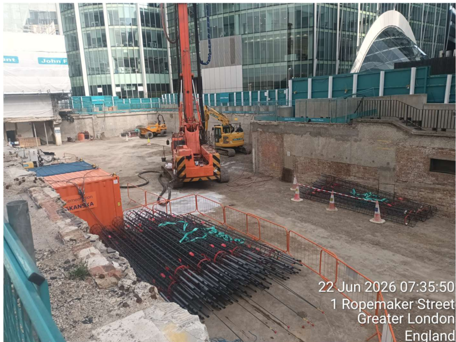
Pile installation works
