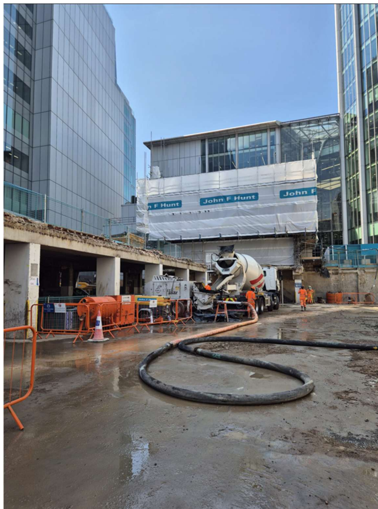
Pile installation works
